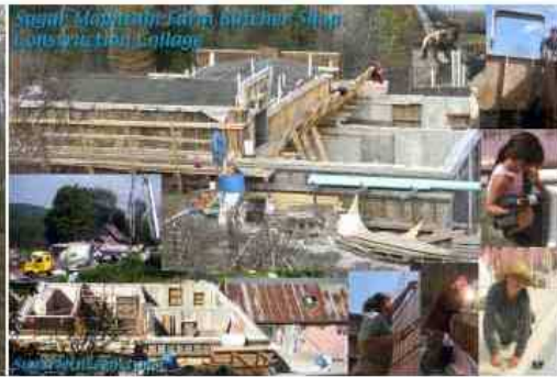
Butcher Shop Construction
